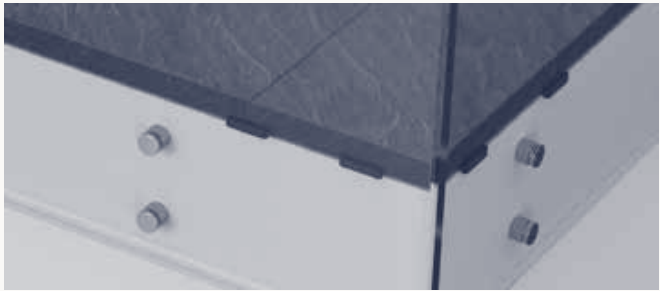
Wall spacer between tiles and glass railing
