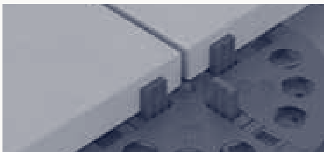
Spacer tab setting the joint between tiles
