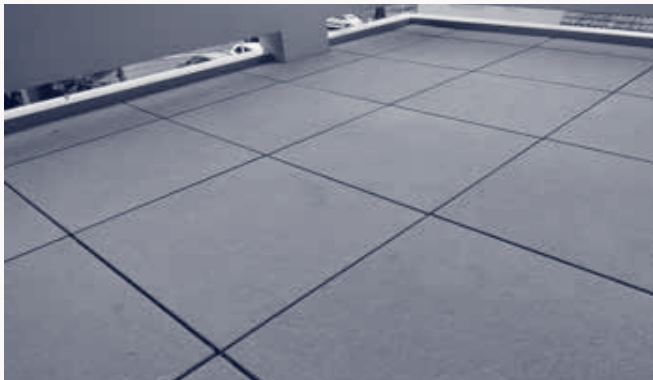
Level, open-jointed finish on a raised floor
