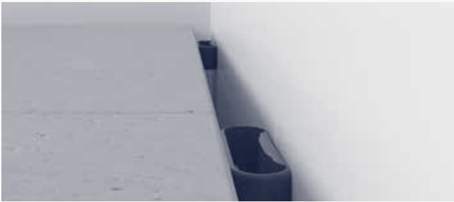
Constant distance between tiles and wall
