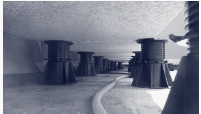
Free void beneath for services and drainage
